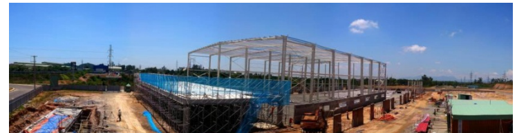
Apple Film Da Nang construction site in May 2014
